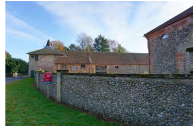
Flint and brick wall to the Maltings site
