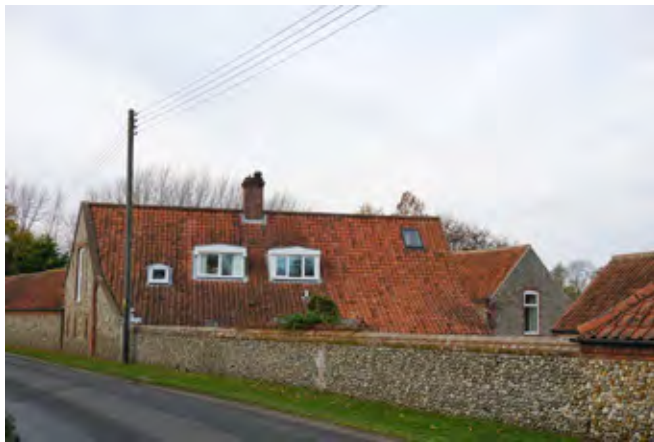
Converted barn at Home Farm
