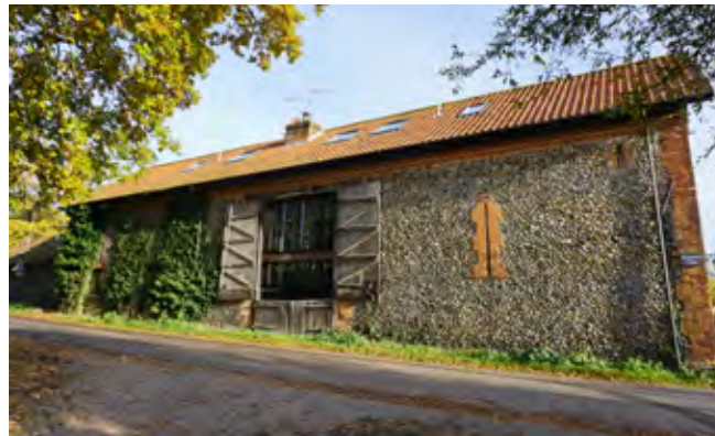
Converted Pigotts Barn on Riverside Road
