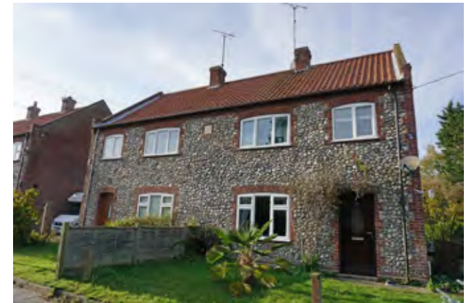
Modern cottages on Riverside Road
