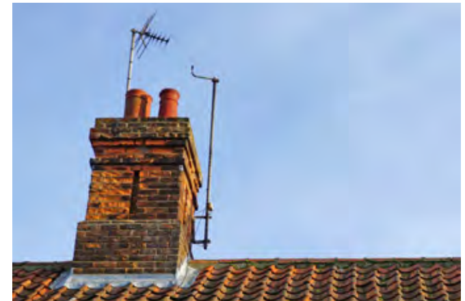
Eroding brickwork on a chimney
