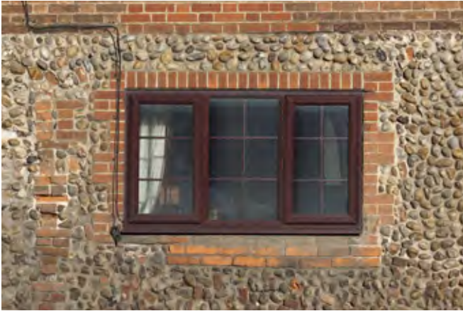
Inappropriate uPVC window
