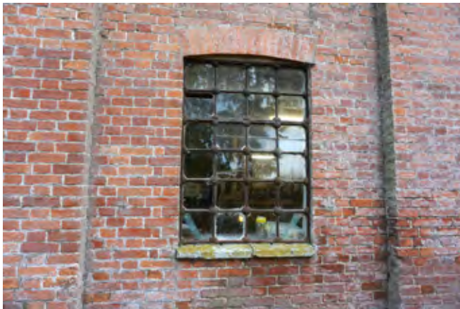
Rusting and bowed window on the mill
