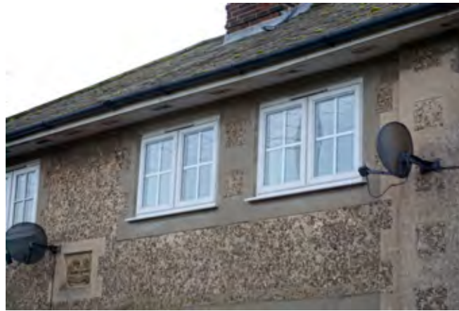
Cement render, satellite dishes and uPVC windows, all inappropriate additions (house currently outside the Conservation Area boundary but proposed for inclusion in section 8)
