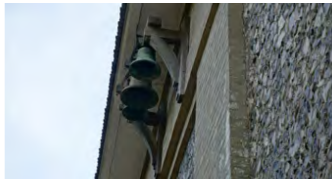
Bells for the Coronation Clock on the north elevation of the former malt kiln
