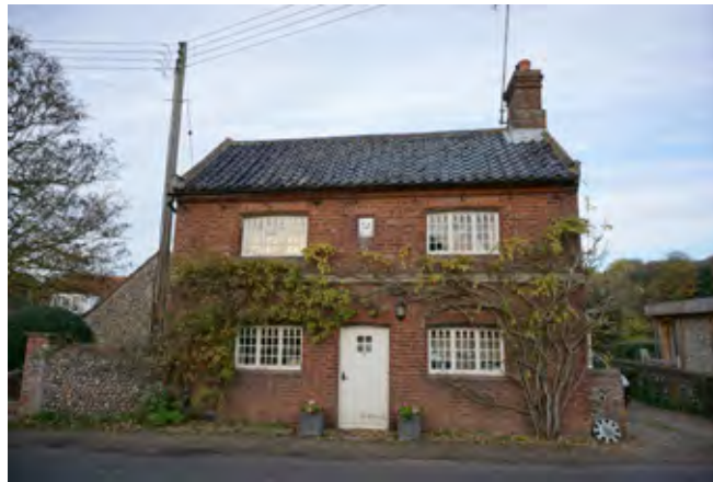
Cottage on Blakeney Road with attractive decorative glazing bars
