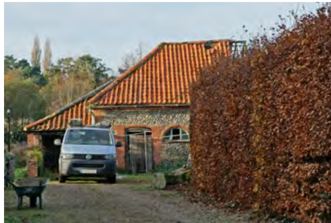
Barn in poor condition with parts of the roof missing
