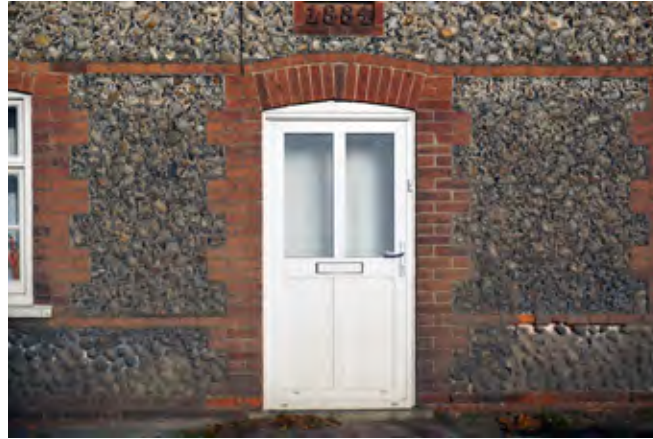
Inappropriate uPVC door
