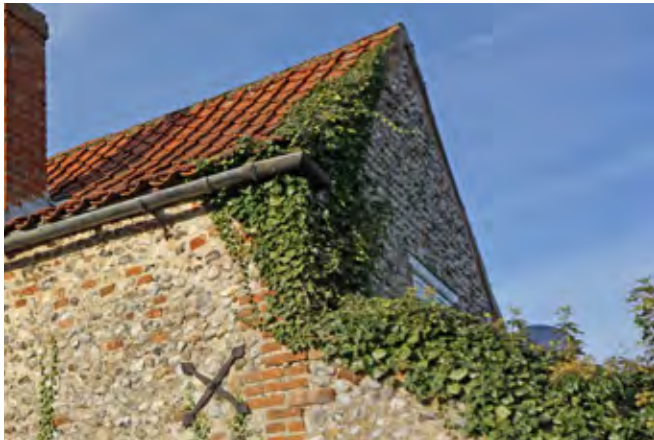
Ivy growth to a building could cause issues with structural integrity and encourage moisture into the building
