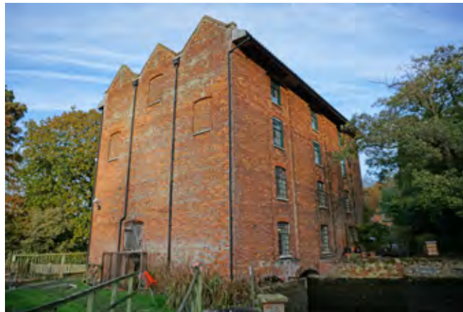
Letheringsett Mill, west and south elevations
