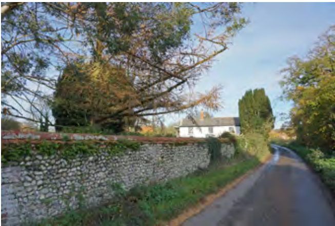
Flint and brick wall on Riverside Road
