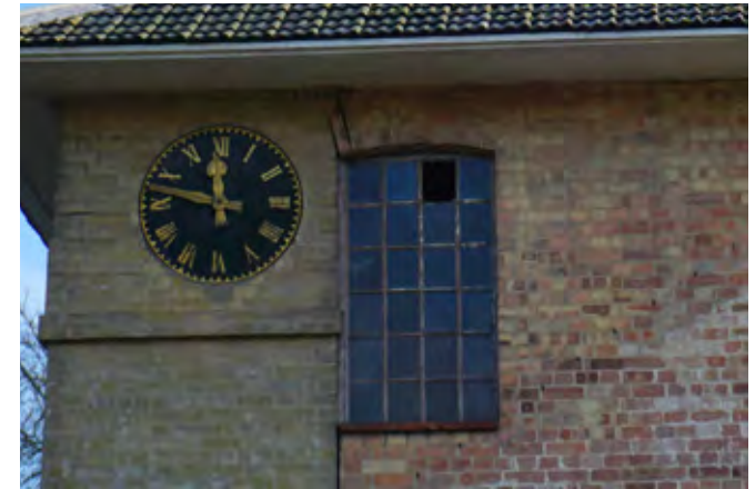
Rusting window frame with glass pane missing
